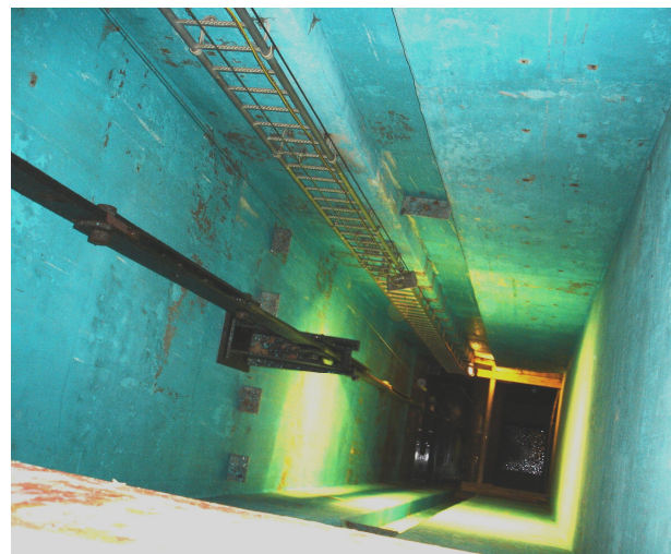
Figure 1: View into the duct of the slide gate chain.
