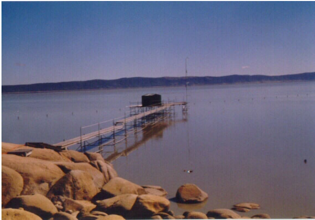
Figure 5. A view of the observation platform from the shore. The elevated walkway can be seen in the foreground, with the accommodation module visible on the platform.
